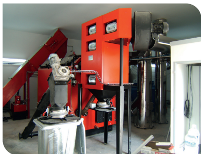
> Chaudière bois - Scey-sur-Saône
